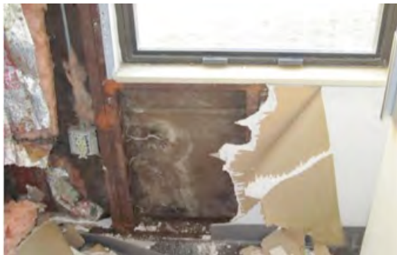
Step 1: Remove Major Portions of Existing Framework and Veneer
