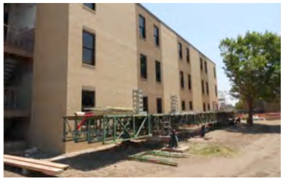
Step 4: Reapply Exterior Veneer
